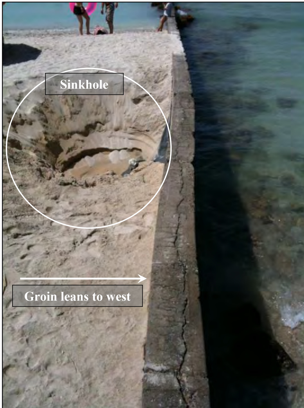
Figure 3-6 Looking seaward along the crest of the groin, from the Sheraton seawall.
