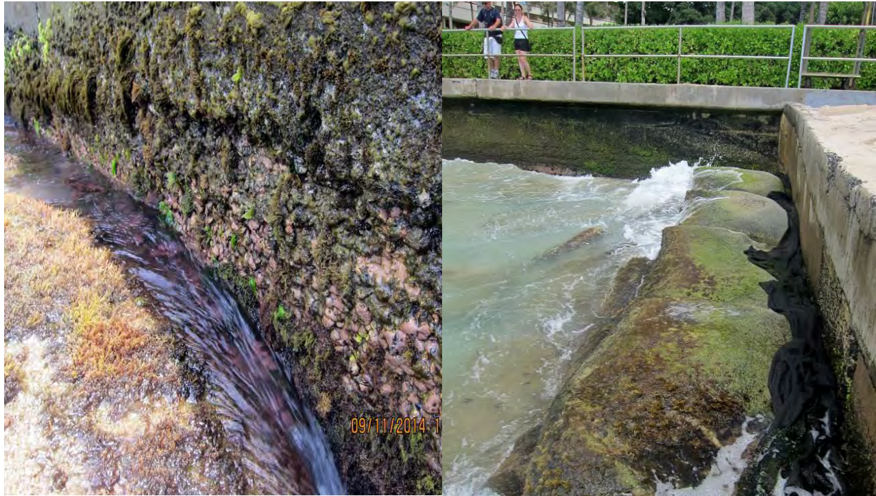
Figure 5. The inner groin is coated in macroalgae and crustose coralline algae (CCA; photo at left). Several stacked sand bags, with macroalgal and cyanobacteria; growth, lie along the base of the west side of the groin (photo at right).
