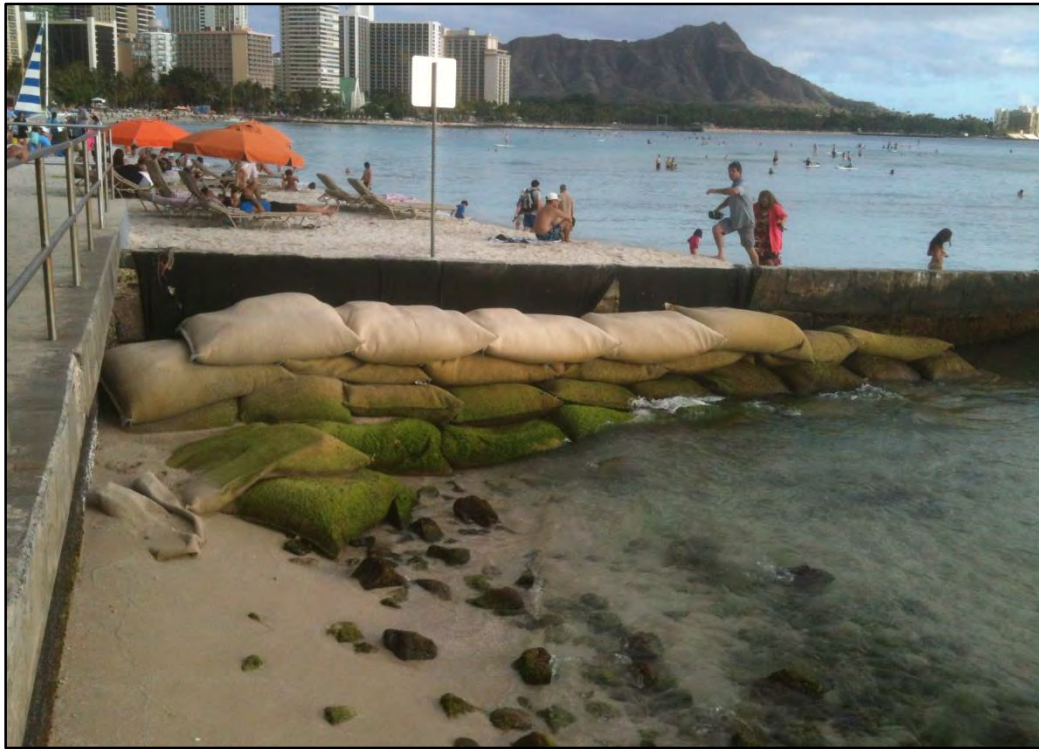
Figure 3-7 ElcoRock sand bags one month after placement (photo date January 21, 2013)
