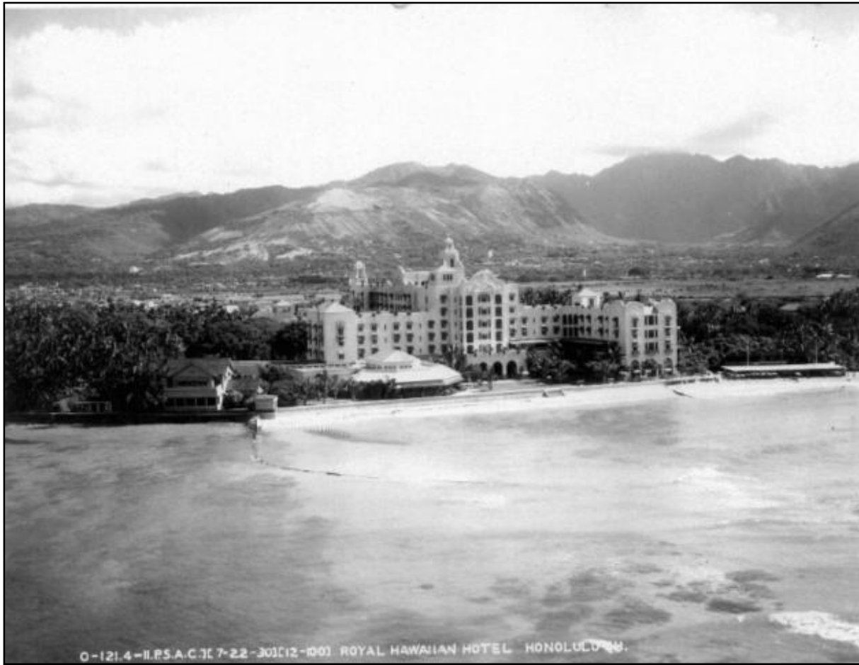
Figure 3-1 1930 historic photograph of the Royal Hawaiian Groin. Rocks are placed on the west side of the structure, near the shoreline, to stabilize the stacked concrete block structure.
