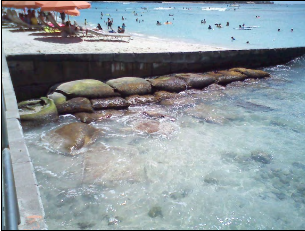
Figure 1-2 Photo of existing groin (September 25, 2014)
