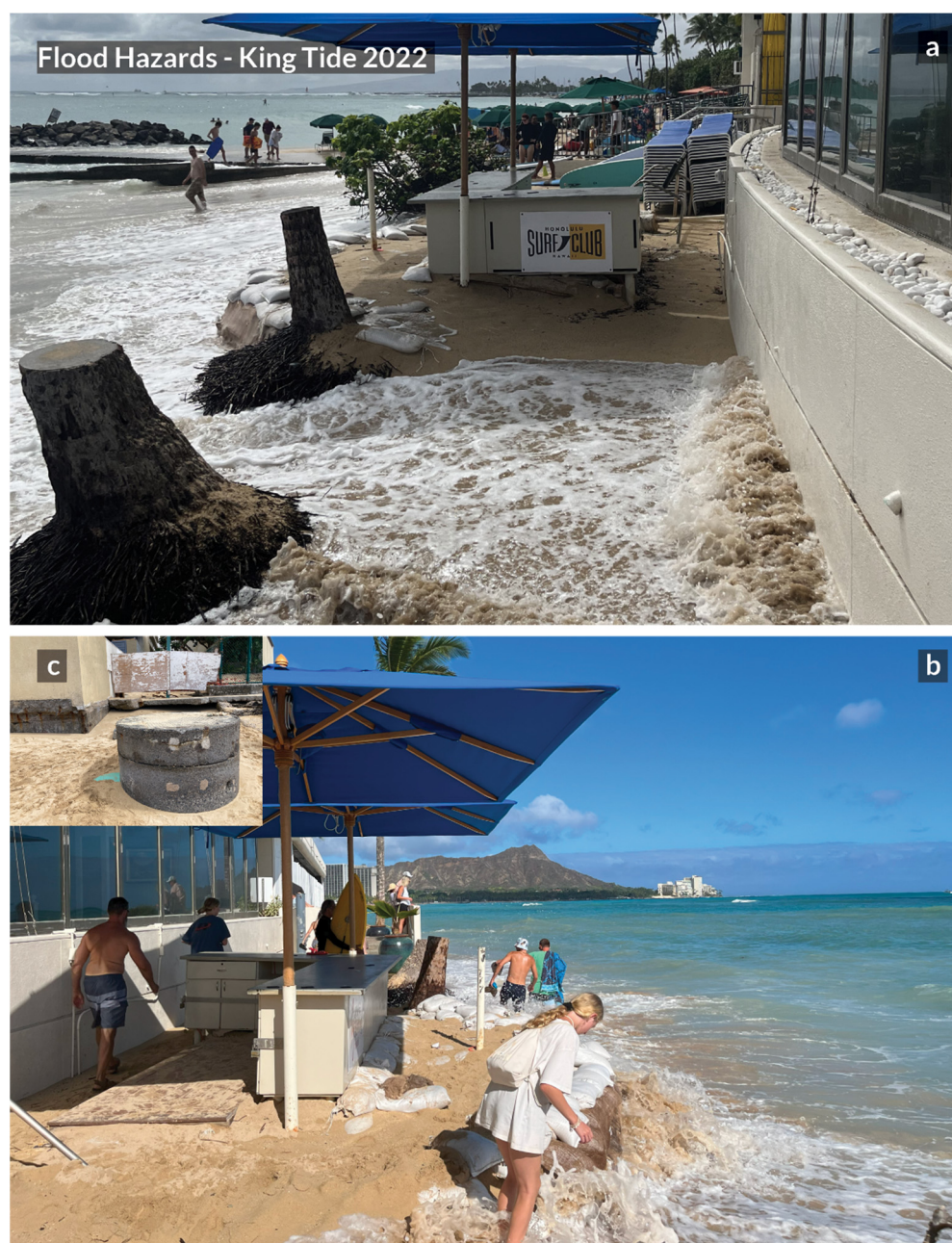
Figure 1. Images in summer 2022 during a king tide event at high tide showing (a) high wave run-up and loss of vegetation, (b) inundation of the beach and building edge, and (c) exposed infrastructure. Credit: Eric Teeple, Melanie Lander, and Wendy Meguro.
