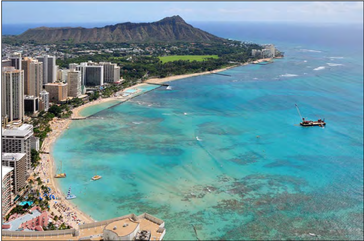
Figure 10: Beach nourishment at Kūhiō Beach showing the nearshore dredging system and dewatering basin onshore. 2012.
