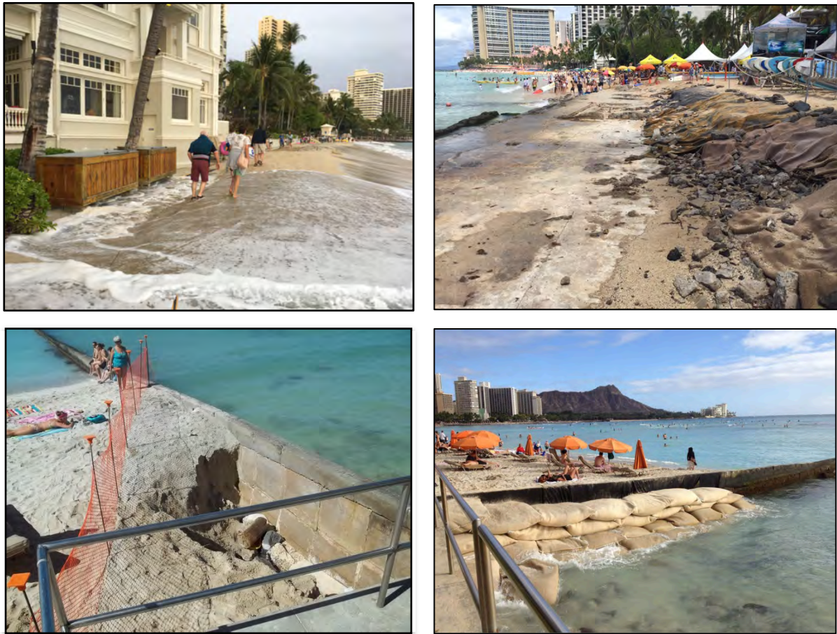
Figure 6. Examples of beach erosion, Inundation and structural failure in Waikīkī.
