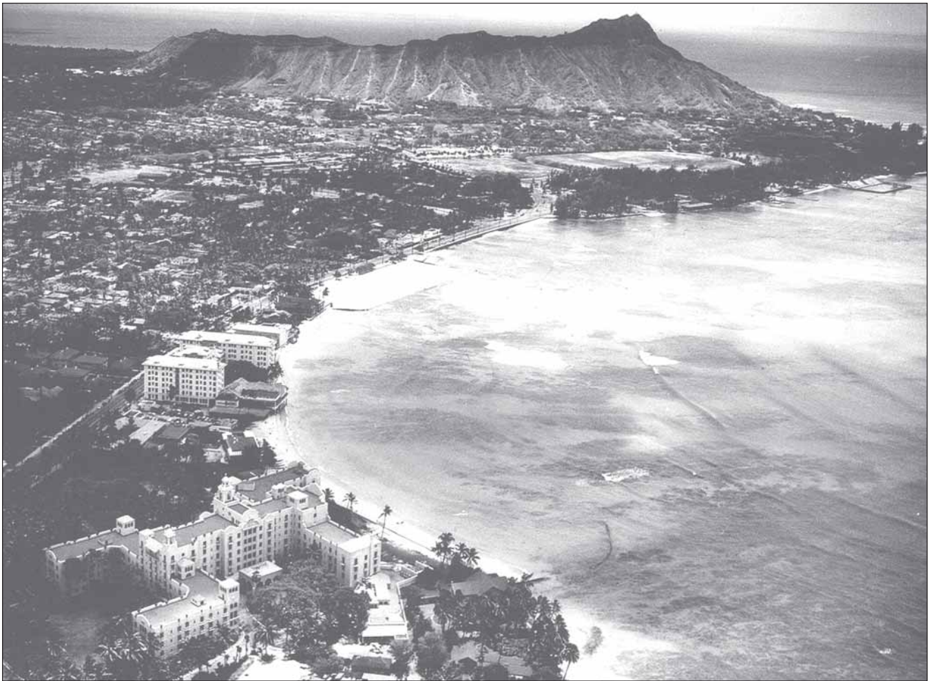
Figure 11. Aerial photo, circa 1940, looking toward Diamond Head; Royal Hawaiian-Moana Hotels Beach (curved groin near bottom); Kuhio Beach; “crib wall” breakwater; seawall along section of Kalakaua Ave.; Natatorium in distance at top right. (By Anon.)
